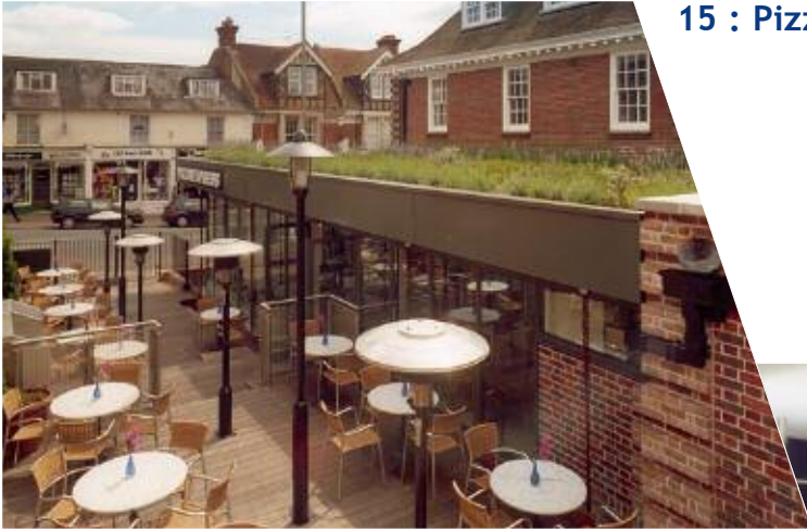
Pizza Express : Uckfield : External Facade
